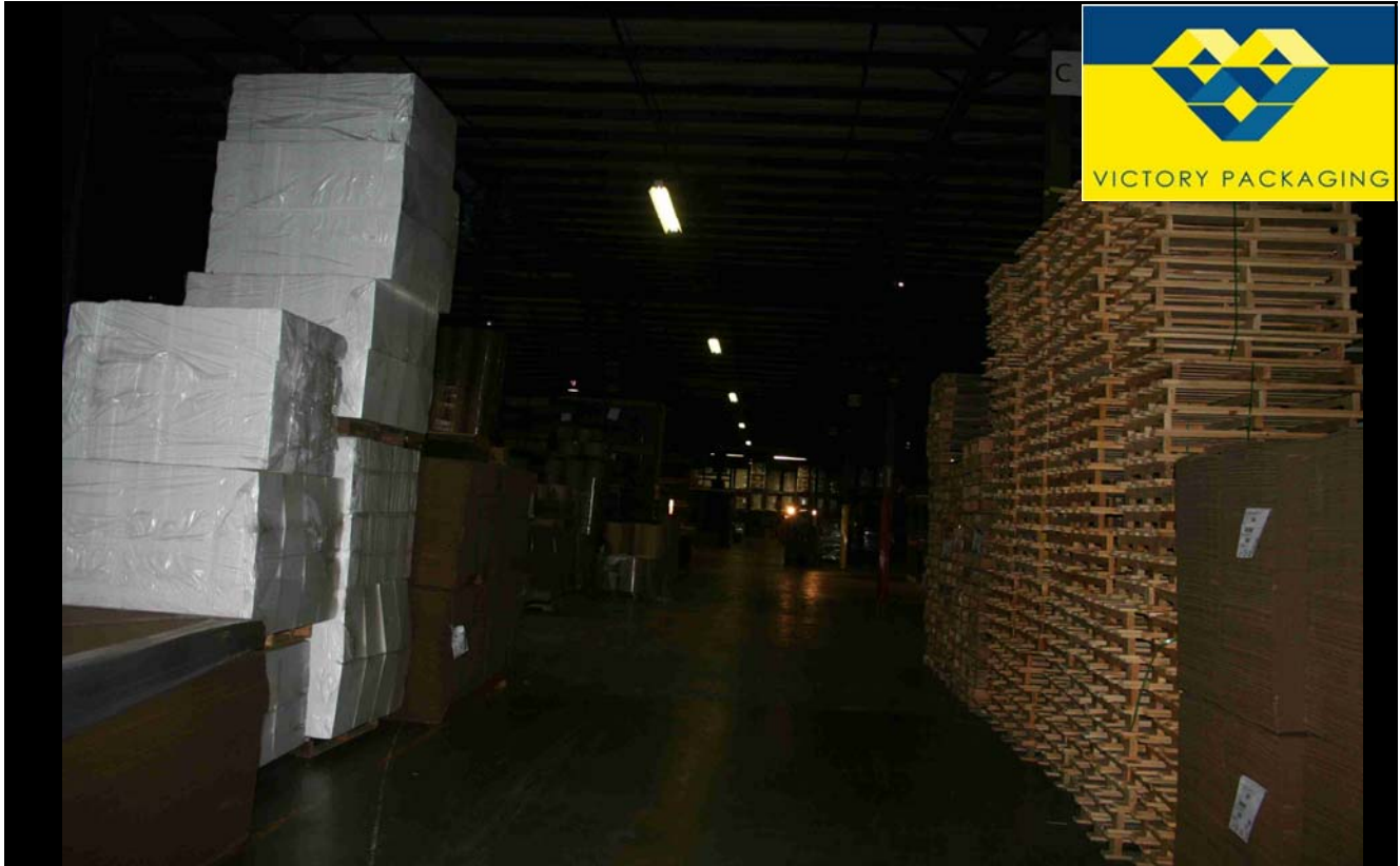
Before – 2 Lamp T-12 Strip Fixture with Magnetic Ballast
